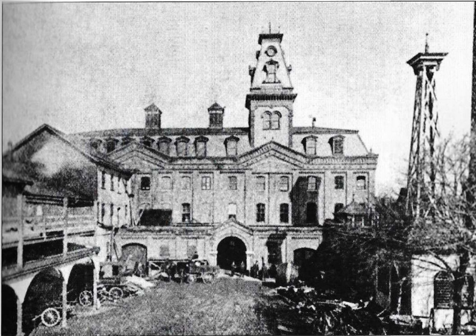
HARTMANN & FEHRENBACH BREWERY, c. 1890. H&F undertook its most significant capital upgrades ever in 1888 when they added a 125-foot-long four-story structure, housing a new brewhouse and cold-storage facility. In addition, the old lagering vaults were retrofitted with a refrigeration machine. The Frederick Wunder–designed building increased the brewery’s annual capacity to 75,000 barrels, which, at that time, made it the largest and best-outfitted brewery between Philadelphia and Baltimore, Maryland. (DHS.)
